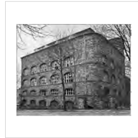
Fábrica Goeritz, Chemnitz (1925-27)
